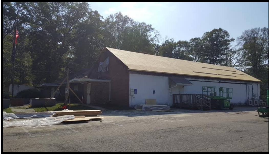
The new roof work in place
